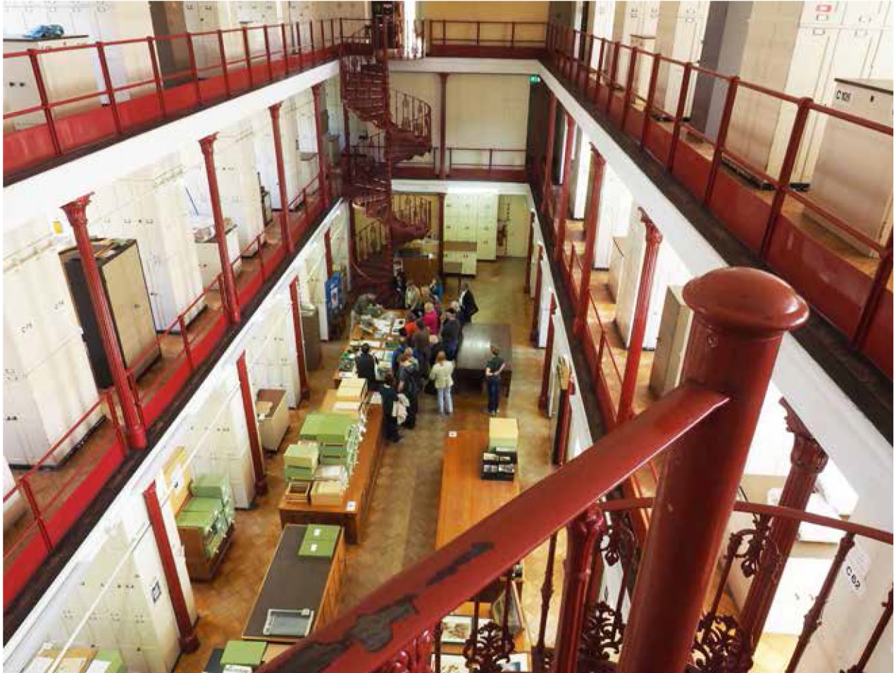
Fig. 9. The Herbarium of the Royal Botanic Gardens, Kew, interior of what is now Wing C. Built in 1876–1877 for storage and work with herbarium specimens over three floors, the upper two galleried on iron columns. The design maximised admission of natural light as gas-light presented a serious fire hazard. In 1903 the building was stripped of its elaborate ironwork and wooden panelling, fire-proof concrete floors laid, and the galleries widened. The original interior can be seen in an early photograph reproduced in R. Desmond's history of Kew (Desmond 1995: 248). The building was added to the oldest part of the present herbarium complex, the Hunter House, to hold the rapidly growing collections. At the appointment in 1841 of the first director of the Royal Botanic Gardens, William Hooker, there was no official herbarium at the gardens. Hooker made his own collections available to staff and visitors on the ground floor of the Hunter House; the collections grew so quickly that this purpose-built wing was added in 1876–1877. The next wing, currently Wing B, also with three floors, was added in 1902. Wing A, with four floors, was added in 1932. A fourth Wing D closed the quadrangular courtyard in 1969. A basement with compactors was added under the quadrangle in 1990, and a fifth Wing E was added in 2009. Photo and information kindly provided by David Goyder, Kew.
